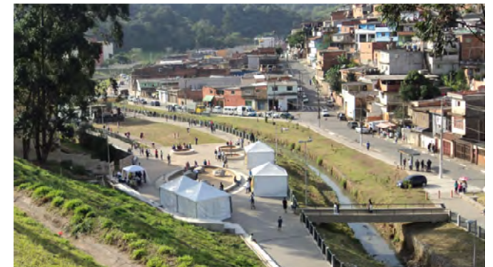
Figura 10. Parque linear Córrego do Canivete, Sao Paulo, Brazil (Ana Beatriz Silva Lima, Municipal Secretary of Green Areas and the Environment of São Paulo, 2012).
